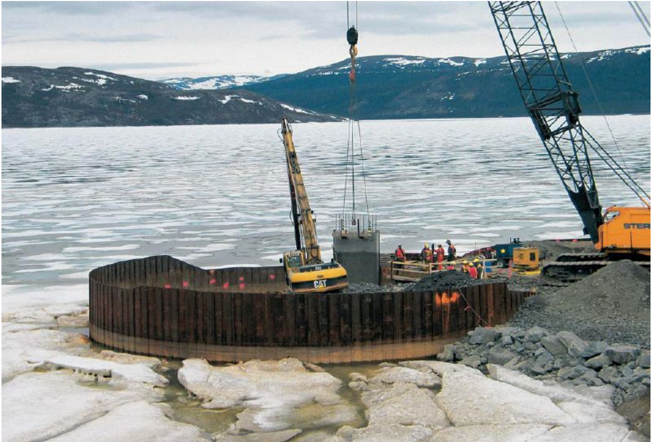
Figure 12 - Sheet Pile Installation in Arctic Environment
