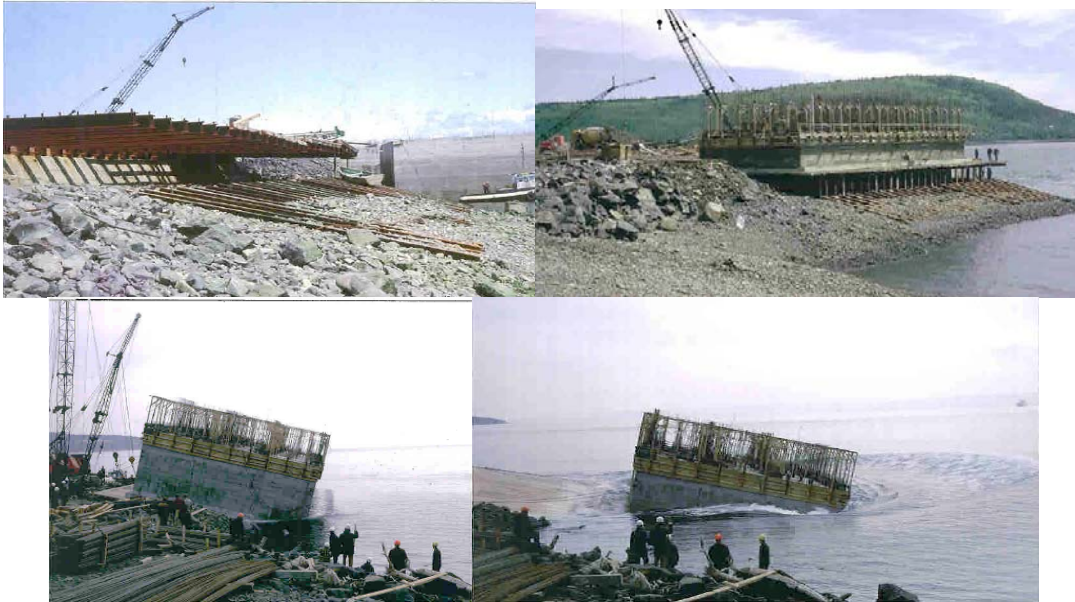
Figure 15 - Concrete Caisson Construction and Launch
