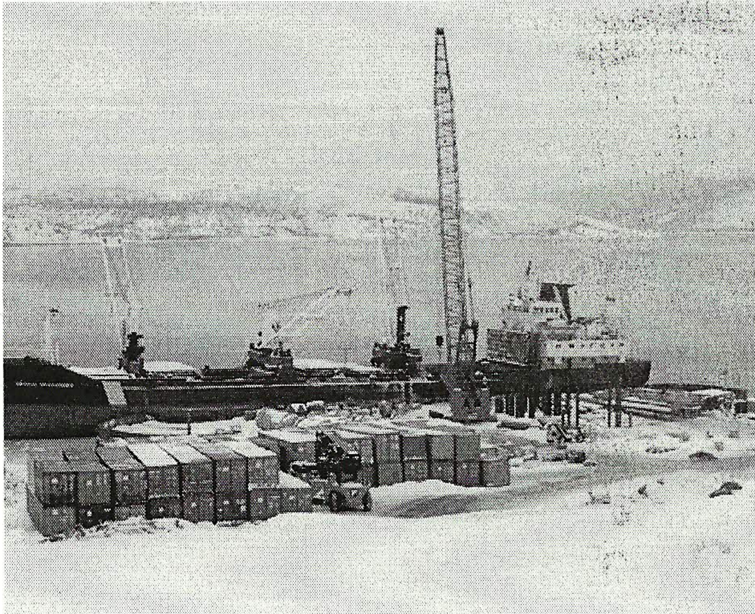
Supply ship docking at the sheet pile wharf in Voisey's Bay
